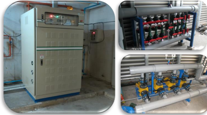
Ozone for Cooling Tower, ESPLANADE
