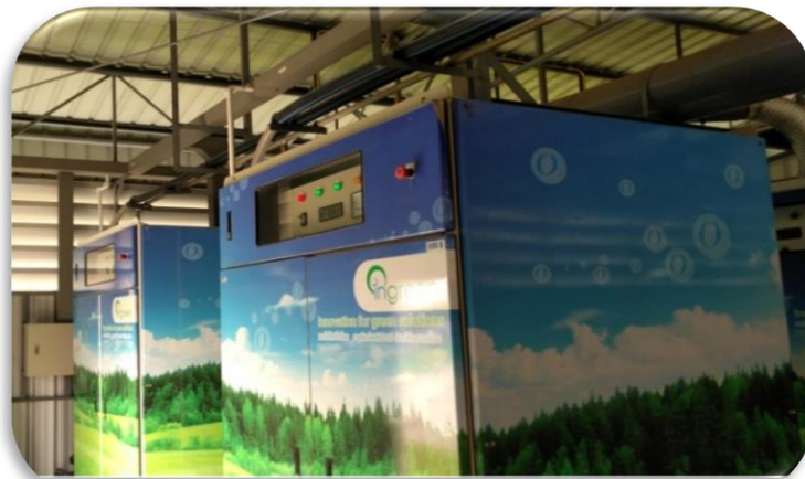
Ozone System, PWA - Chachoengsao
